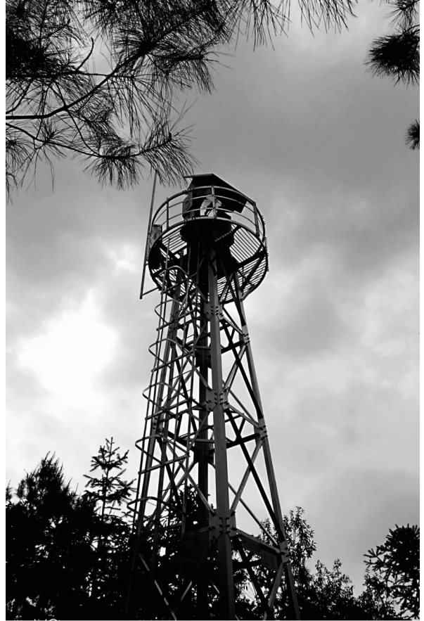
图7 架设在长沙机场铁塔上的子阵1 Fig. 7 No. 1 subarray on the top of an iron tower at Changsha Airport
